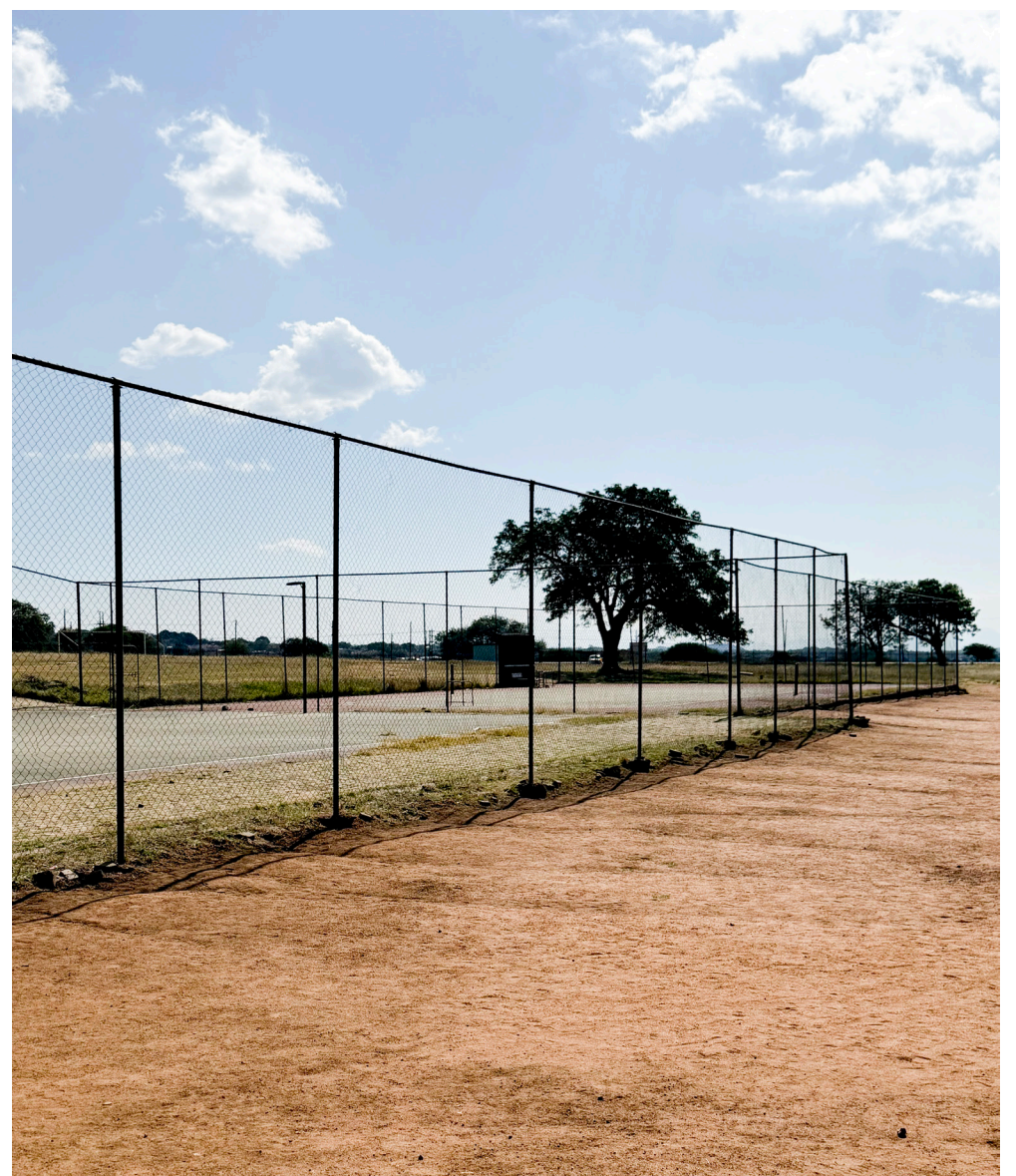
Marishane community constructed a tennis and netball court.
